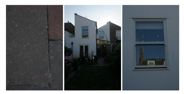
Turning to the main building, all of the external surfaces are rendered which can tend to be a short term solution as inevitably rain after only a couple of years will tend to soil the façade if not allowing water behind which will then freeze and disturb the surface but at the moment it appears to be in good condition although there is some aberration to the paint above the first floor window to bedroom 3.
