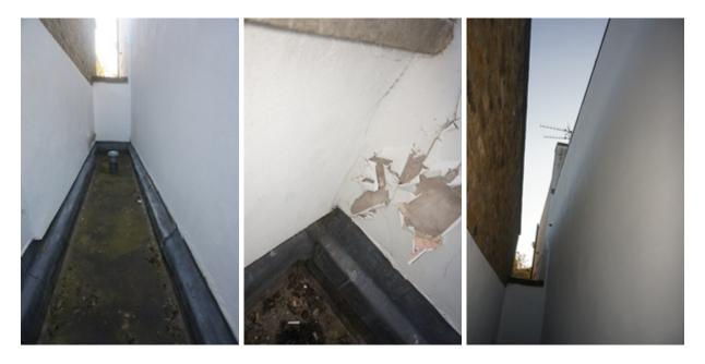
To the base of the render there is a black painted plinth and generally all the rainwater goods appear to be in good order, noting that they tend to splash on top of the respective grates rather than beneath them and noting the manhole<sup>6</sup> cover set approximately 2m from the central glazed panel to the conservatory.
