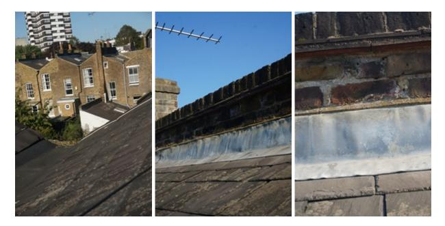
These will continue to slip and require replacement though the roof can be maintained for many years to come, but clearly a decision was made to do this given the relatively new refurbishment to other areas, and the rear roof has been covered with a synthetic tile noting the breather vents set up towards the ridge line which has on the top of it a metal capping with lead detailing beneath dressing onto the synthetic slates; this structure being the gable wall.
