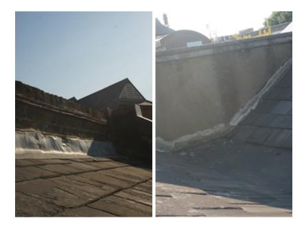
It was possible to inspect the roof and the chimney stack which is in good order, as are the parapet walls on the whole though these should be inspected every two years as inevitably mortar and indeed bricks can be susceptible to frost damage (known as 'spalling') due to their remoteness and relatively high surface area compared with their volume.
