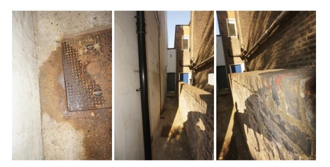
There is an awkward step down to the side alleyway which has a similar concrete ground specification and noting that there is effluent leaking from the far manhole with a pungent smell and obviously this should be investigated.
