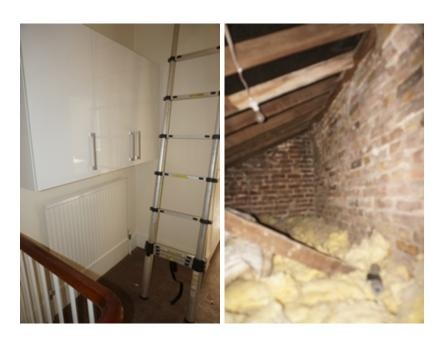
It was noted that, as is traditional, the top of the roof is held up by a timber wall plate which sits on corbelled brickwork which would not comply with Building Regulations but is thought to be quite adequate and there is at the centre height a purlin which also has intermediate supports.
