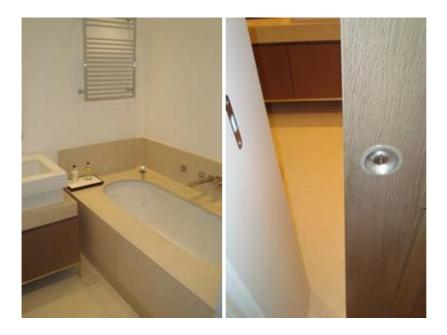
The sliding door to the bathroom requires easing and is very heavy. It is also difficult to open given the recessed type of ironmongery.
