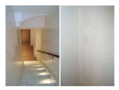
Photograph of stairs down to basement noting that there is some water ingress to the polished plaster and it is believed that this is to be replaced along this wall.
