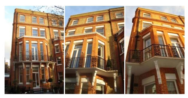
With regard to the stone balcony to the rear (at first floor level) this appears structurally sound – there are no indications of any distress and it is supported by 6 buttresses.
